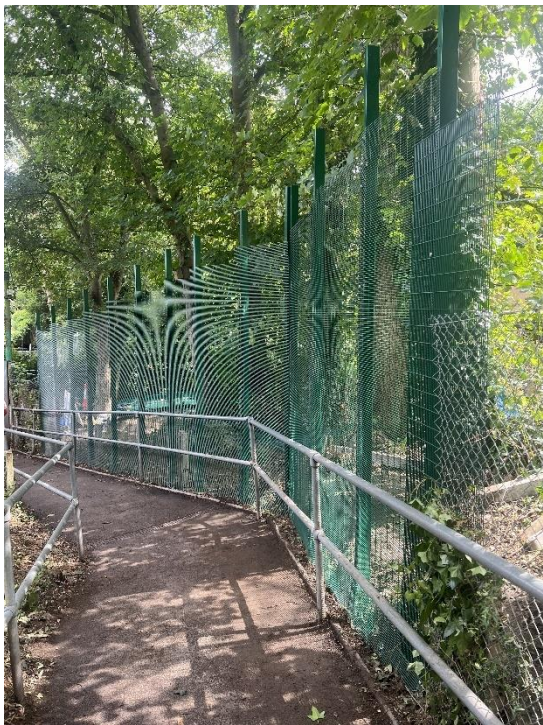
Figure 6 - External view of 3m inner skin installation.
