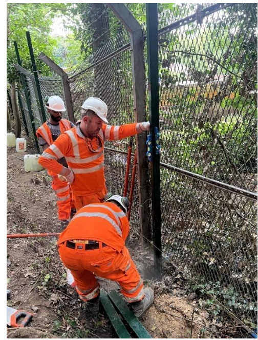
Figure 22 - Installation of posts along the 'yellow' section
