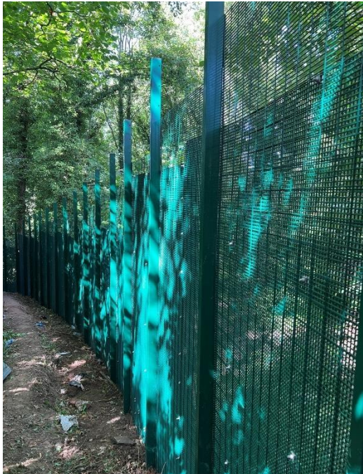
Figure 27 - Internal view of double skinned fencing along the 'yellow' section.
