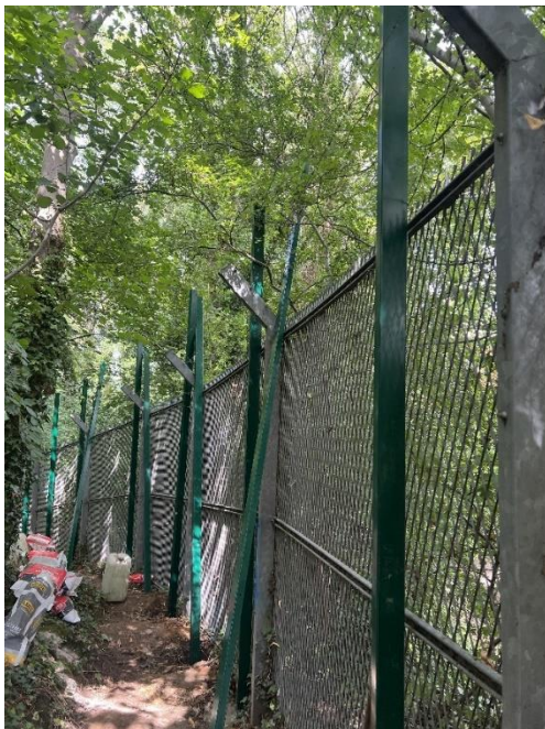
Figure 21 - Posts and postcrete loaded out at each hole ready for installation.
