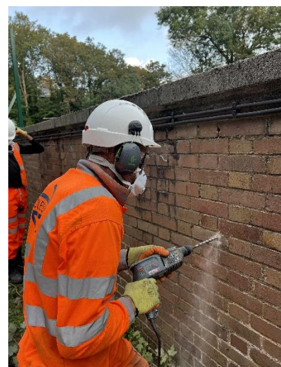
Figure 40 - Drilling 14mm holes for resin fixing.
