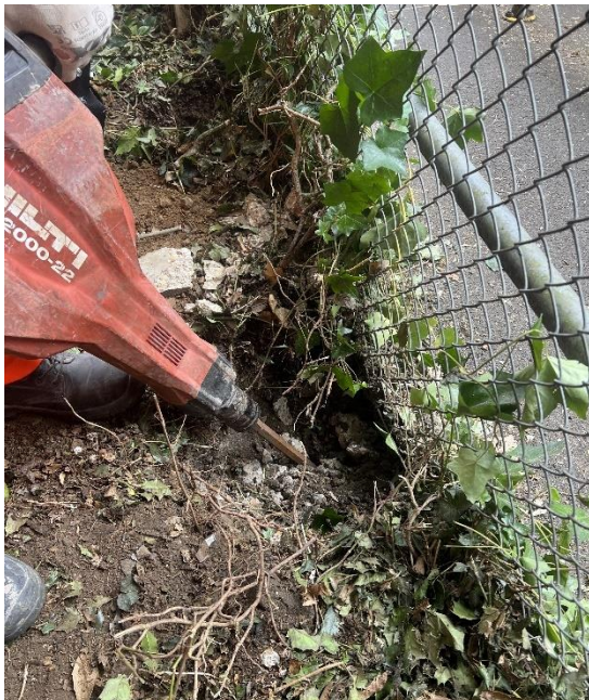
Figure 4 - Breaking out concrete underlay to pathway obstructing post excavations.
