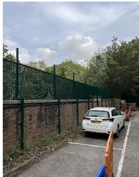
Figure 44 - Prefabricated double skin panels to avoid working at height.
