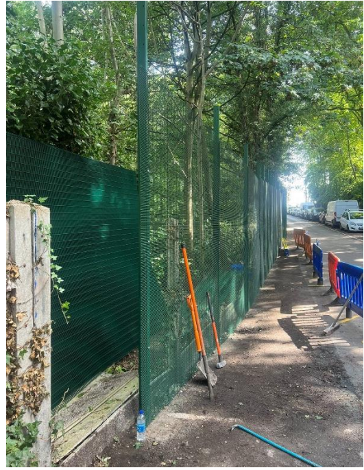
Figure 34 - Car park boundary fencing single skinned and existing concrete panels removed.
