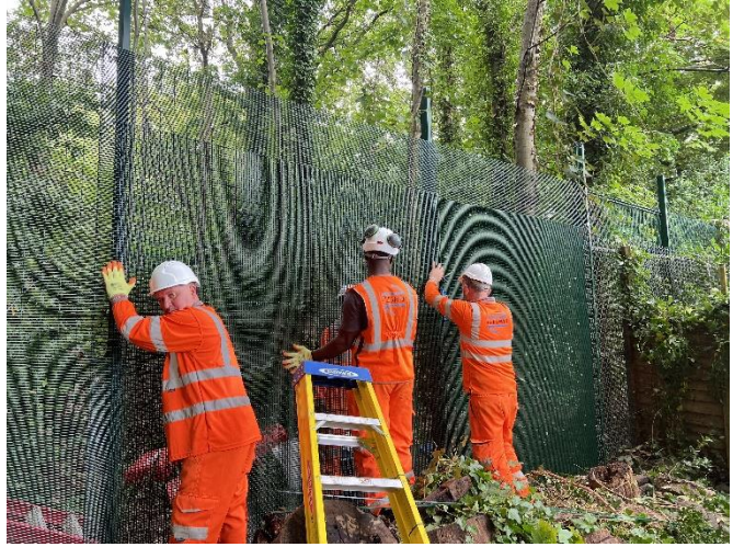
Figure 24 - Double skin resumed once fencing extended beyond the garden of No. 87 Priory Gardens.
