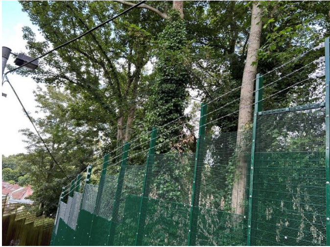
Figure 8 - Double skinned panels finished with 3 strand barbed wire topping.
