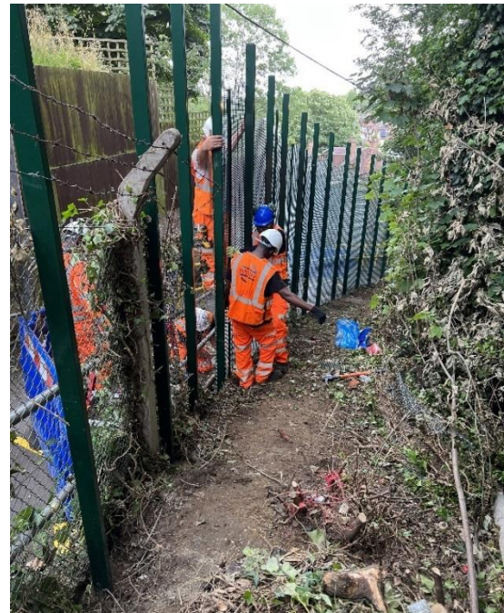
Figure 5 - Installation of panels along the 'Blue' section
