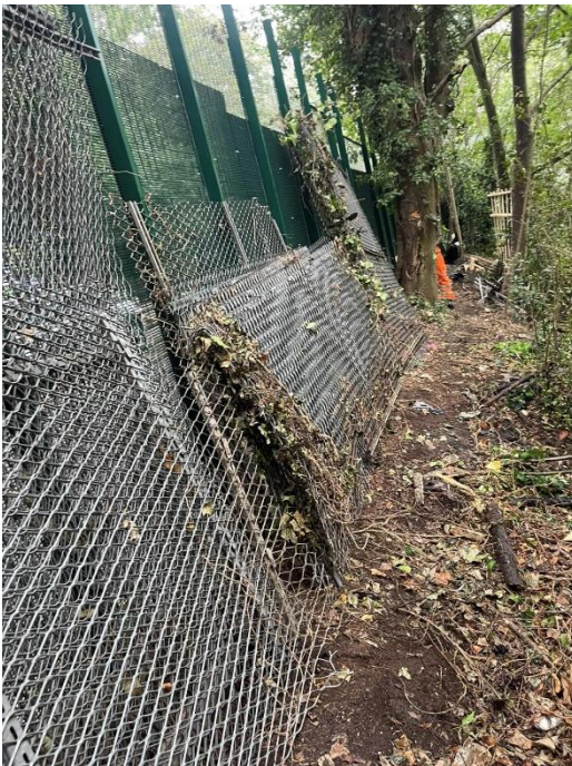
Figure 35 - All redundant scrap and waste material piled in one location ready to be loaded onto the flatbed truck.
