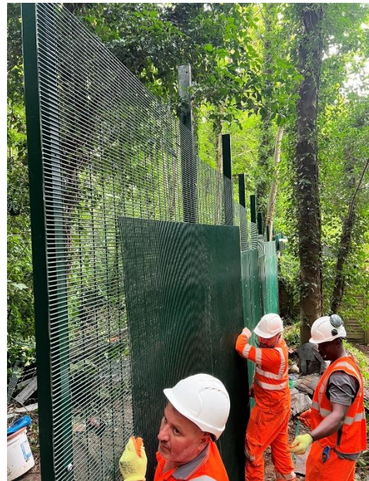
Figure 26 - Installation of double skin panels continued
