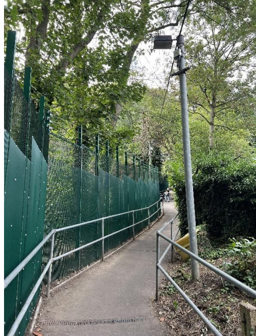
Figure 9 - Double skinned panels finished at the bottom of the pedestrian pathway.
