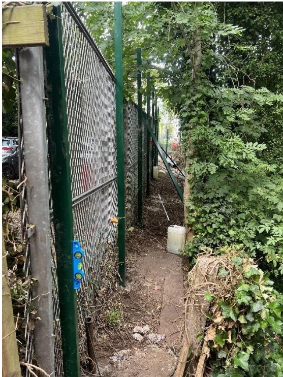
Figure 10 - Uneven ground conditions to working side of boundary.
