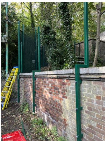
Figure 39 - Dog legged SHS posts resin fixed to car park perimeter wall.
