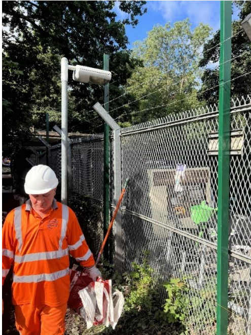
Figure 19 - Existing rhomboidal mesh panels and crank posts removed.
