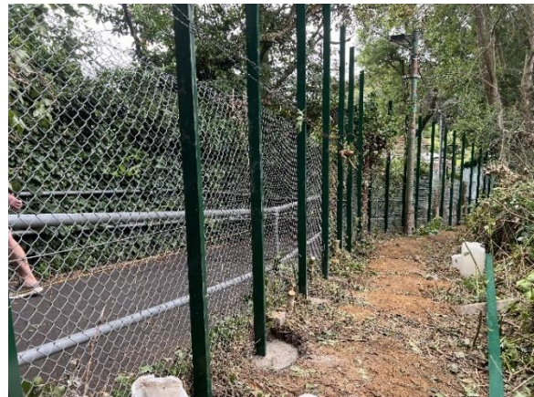
Figure 3 - Posts installed at 1m c/c to accommodate severe gradient.
