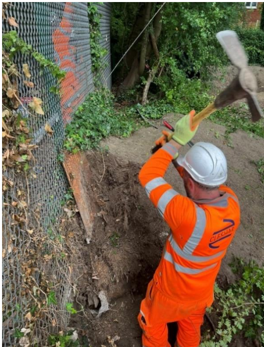
Figure 29 - Reducing raised external ground levels to install new fence panels.
