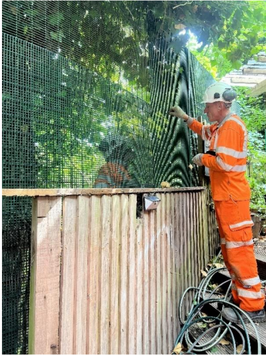
Figure 17 - Installation of double skin panels tight to decking of pub garden.
