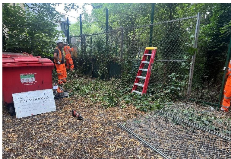
Figure 12 - Removal of existing rhomboidal mesh panels to pub car park
