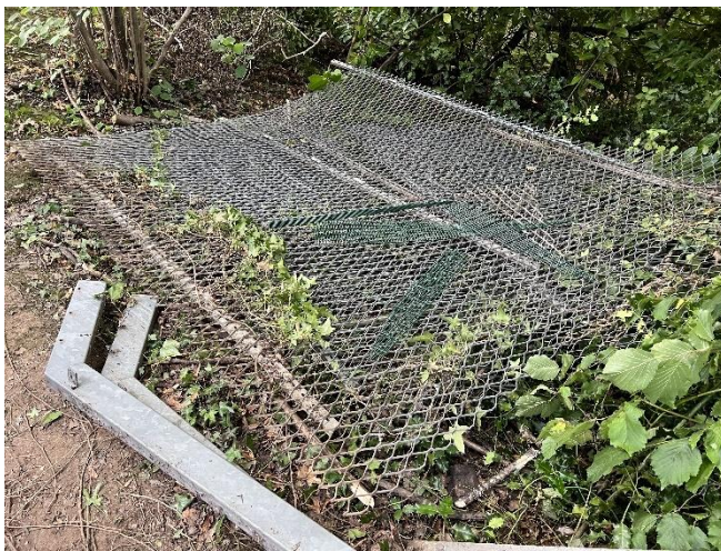
Figure 25 - Removal of existing rhomboidal mesh panels and cranked steel posts.
