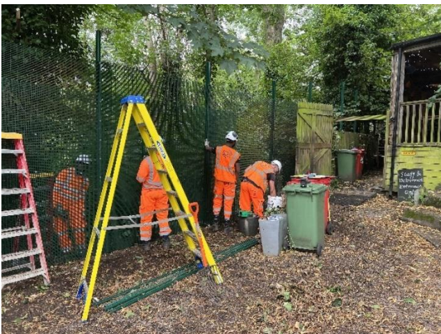
Figure 15 - Installation of double skin panels along pub car park boundary
