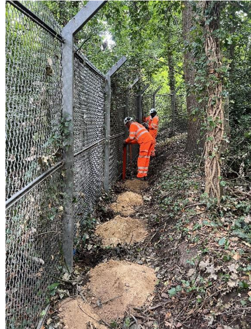
Figure 20 - Excavated piles of strong ballast strata.
