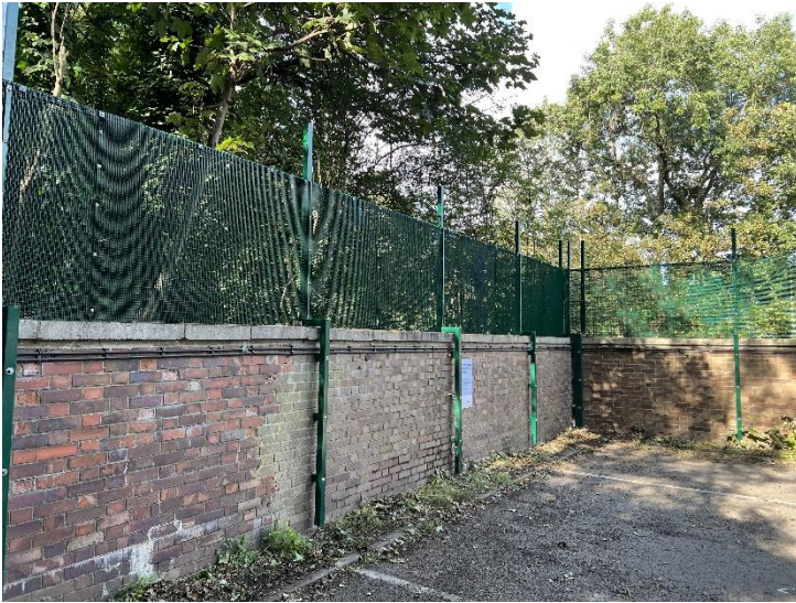
Figure 41 - Carpark fencing double skinned.
