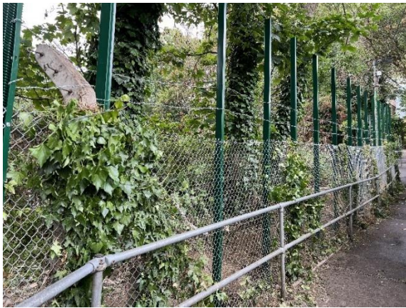
Figure 2 - Existing Chain-link Fencing removed.
